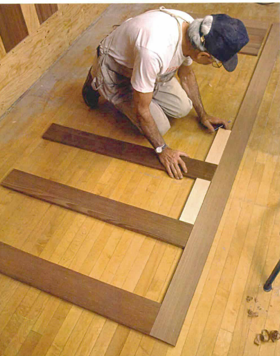
Old redwood sees the light of day. As Karpilow uses his brad gun to attach thin redwood panels to their nailers, the color and pattern of the redwood start affecting the room (photo above). Plywood strips between redwood panels (photo right) provide backing for the frame and trim pieces.
