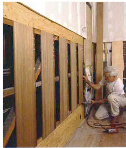
Old redwood sees the light of day. As Karpilow uses his brad gun to attach thin redwood panels to their nailers, the color and pattern of the redwood start affecting the room (photo above). Plywood strips between redwood panels (photo right) provide backing for the frame and trim pieces.
