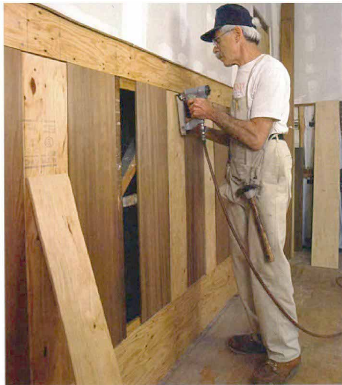
Old redwood sees the light of day. As Karpilow uses his brad gun to attach thin redwood panels to their nailers, the color and pattern of the redwood start affecting the room (photo above). Plywood strips between redwood panels (photo right) provide backing for the frame and trim pieces.
